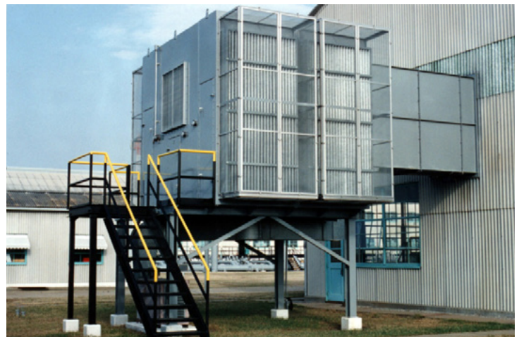
A GTAf 50 retrofit installation for a GE Frame 3 turbine station in Monroe, Louisiana with bug screens, weather louvers, and bypass door.
