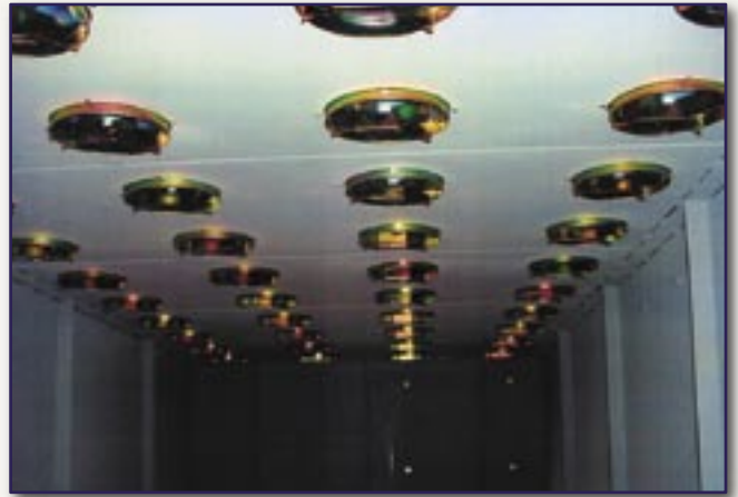
Filter Element Holding Frame Mechanism
