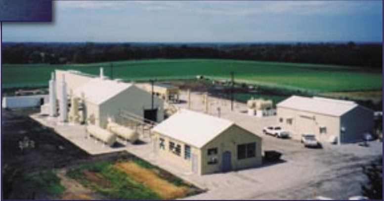
Cooper Bessemer GMW-10-TFT Intake and Exhaust Systems Designed to Meet 60 dBA at 50 ft. From Compressor Building
