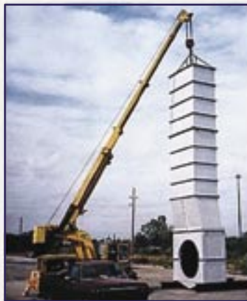
GE Frame 3 exhaust collector and exhaust stack
