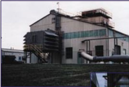
GE Frame 3 barrier type static
