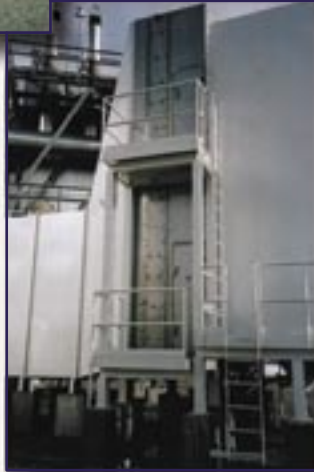
Retrofit of Donaldson self-clean air filter with 90% efficient evaporative cooler
