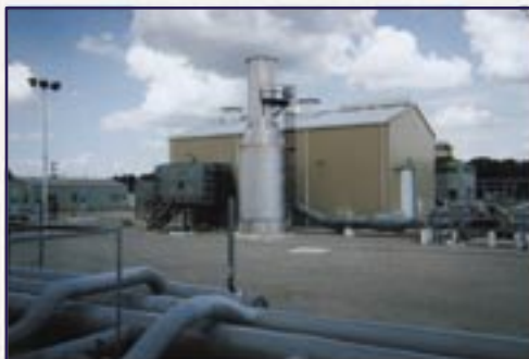
Solar Mars inlet air filter and high performance exhaust silencer
