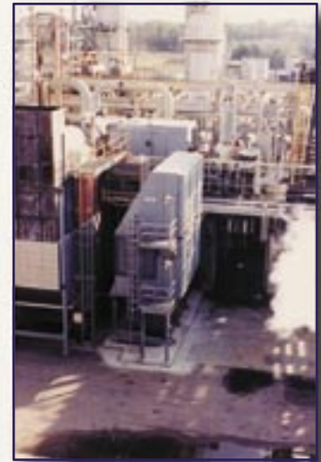
GE Frame 5 barrier type static air filter
