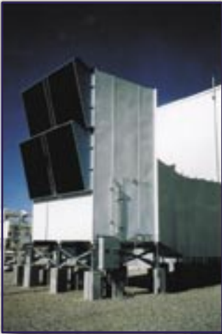
Retrofit of Donaldson self-clean air filter with 90% efficient evaporative cooler
