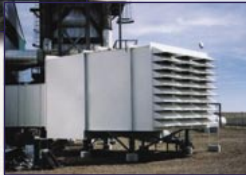
GE Frame 3 self-clean air filter
