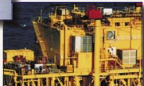
GE LM 2500 off shore gas turbine compressor set inlet air filter manufactured from 316
