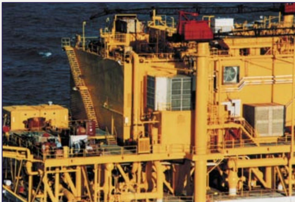
GE LM 2500 off shore gas turbine compressor set inlet air filter manufactured from 316 SS
