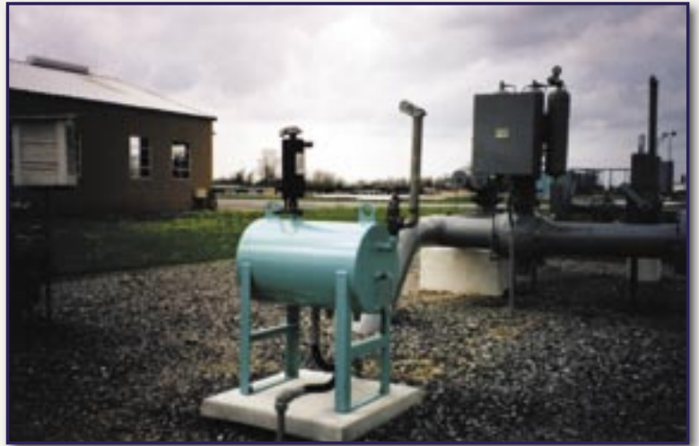
Multi-Connection Gas Over Hydraulic Valve Actuator -15 Gallon Sump
