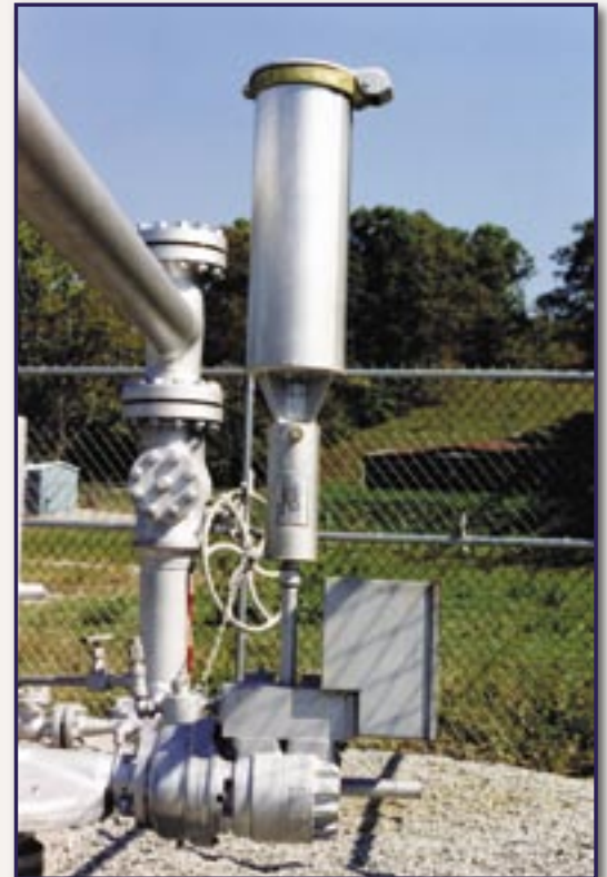
Gas Motor Operated Valve Operator With Vent Mist Extractor Removes 99.8% All Entrained Liquids 6 Microns and Larger With One Gallon Liquid Holding Sump
