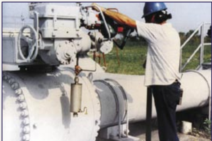
Gas Motor Operated Valve Operator With Vent Mist Extractor Removes 99.8% All Entrained Liquids 6 Microns and Larger.
