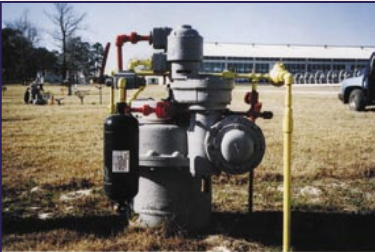
Gas Motor Operated Valve With Operator Vent Mist Extractor/Silencer Removes 99.8% All Entrained Liquids 6 Microns and Larger and Reduces Vent Noise to 85 Dba at 3 Feet
