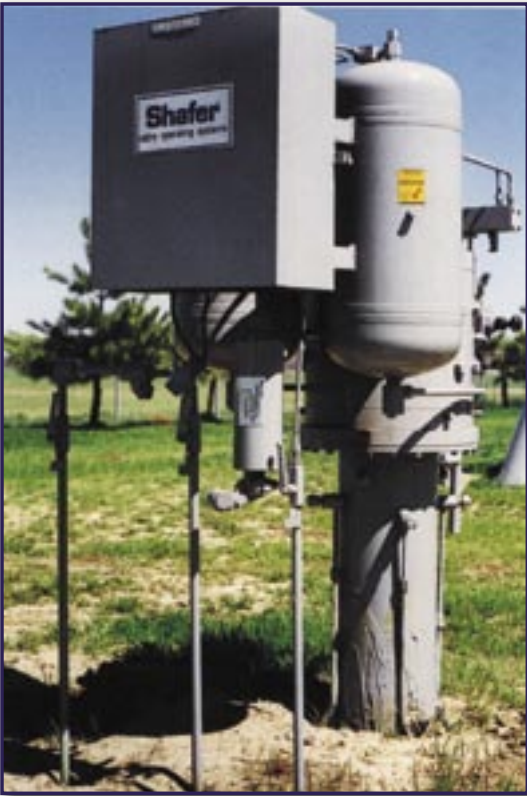
Gas Over Hydraulic Valve Actuator Vent Mist Extractor Removes 99.98% All Entrained Liquids 6 Microns and Larger
