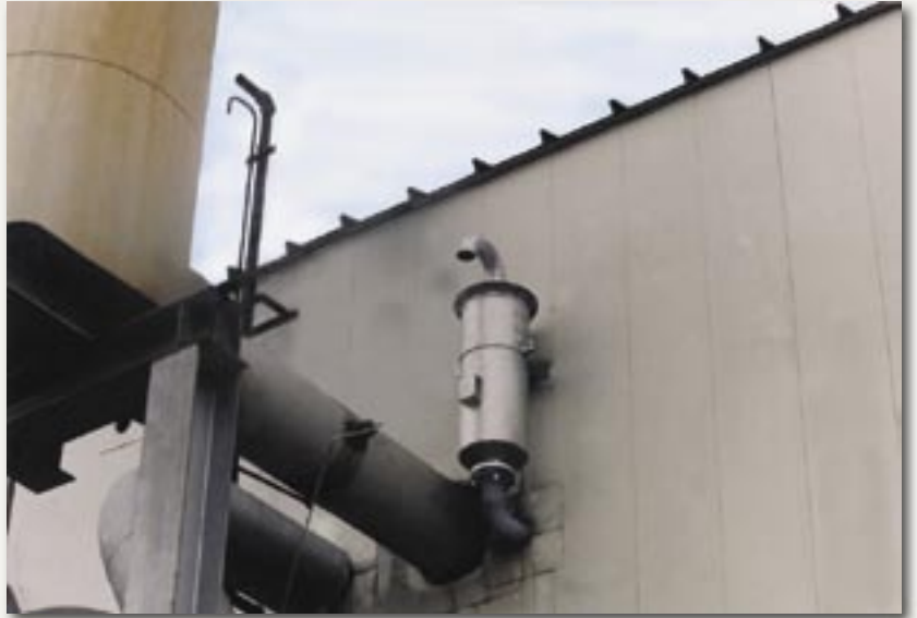
Reciprocating Engine Crank Case Vent Coalescer
