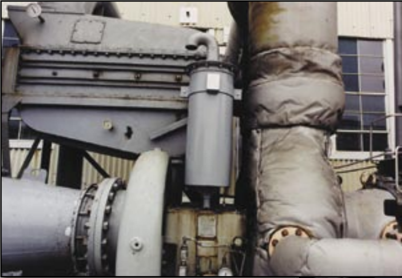
Reciprocating Engine External Turbo-Charger Lube Oil Vent Coalescer
