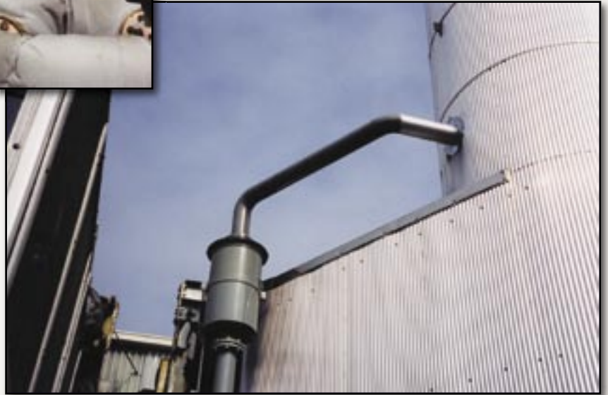
Reciprocating Engine External Turbo-Charger Lube Oil Vent Coalescer
